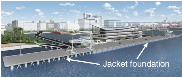
Fig. 2. Jacket foundation for Tokyo International Cruise Terminal.
